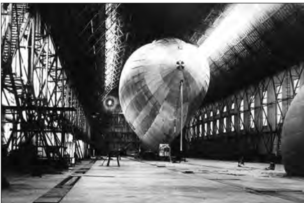
1928 - Italia hangar in Stolp
